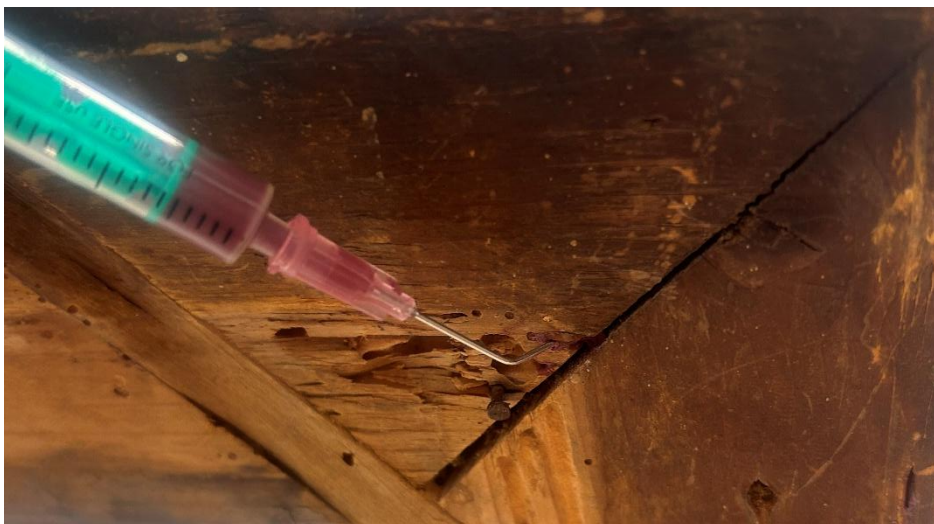
Figure 58 Injection de Plexigum PQ 611
